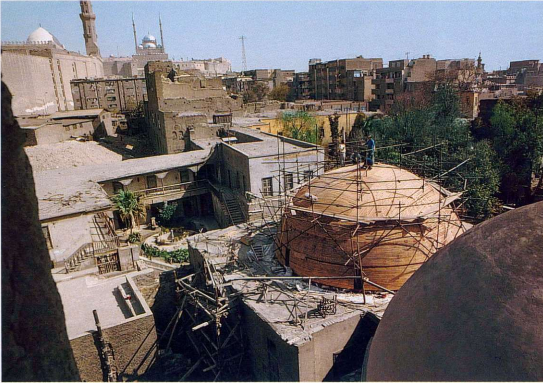
211. The dome of the sama'khana during restoration, with the Citadel and the mosque of Muhammad 'Ali in the background
